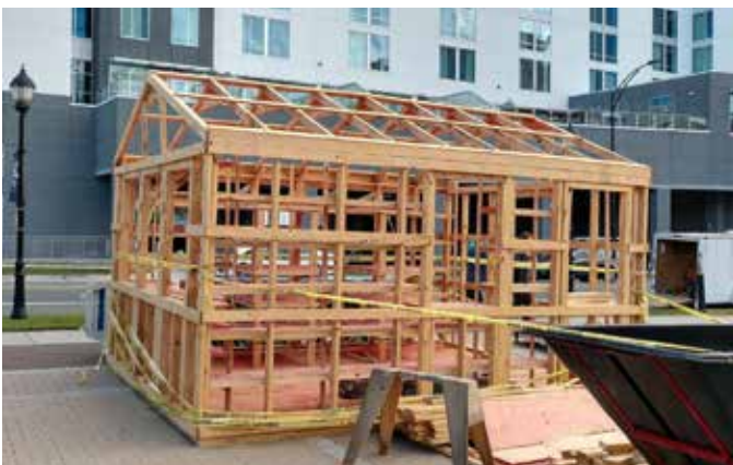
Pyro-Guard® lumber and plywood are used for the construction of outdoor/mall kiosks. Charlotte, NC.
