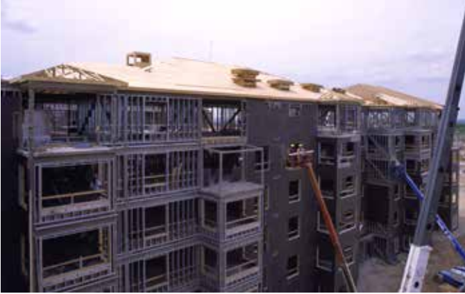
Type II: Pyro-Guard® pitched roof system used as a nail base for 3D architectural shingles in Tulsa, OK.
