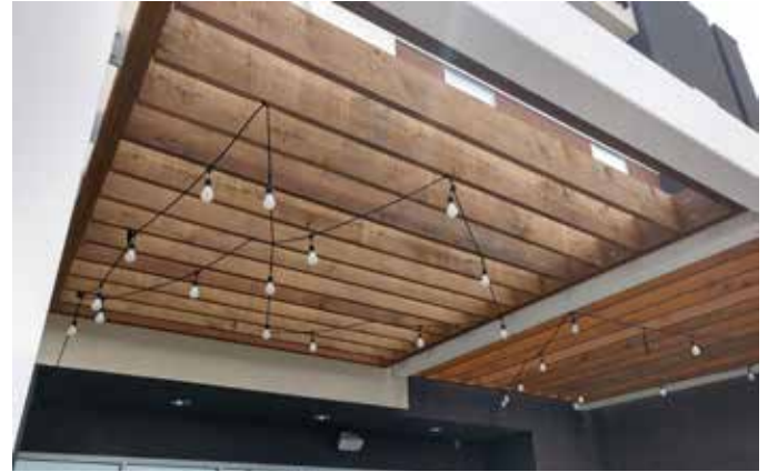
Exterior Fire-X® is often used in weather-exposed applications like this hotel pergola in Denver, CO.
